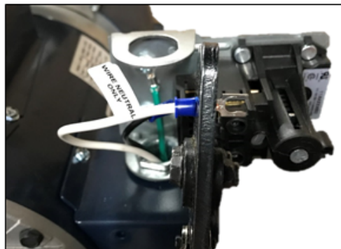
5. Crimp a spade connector onto NEUTRAL wire.
